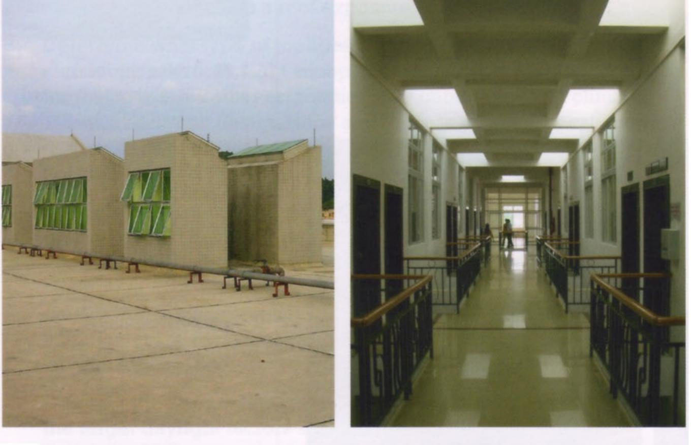
Skylight and clerestory monitors on the roof (left) of the administration building at Guandong Pei Zheng Commercial College in Huadu, China; resulting toplighting distributed by light wells (right) provides illumination for four floors along a circulation corridor.
