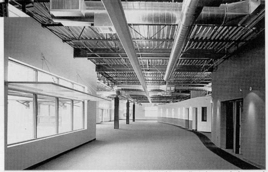
Daylighting provides most of the ambient lighting in the building. Tall windows on the long south side, combined with interior light shelves, allow daylight to penetrate deep into the open office space.
